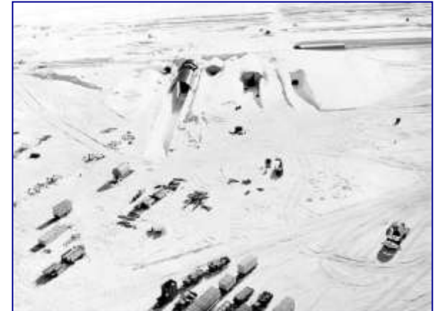
PM-2A: Assembled at Camp Century, Greenland. World's first portable plant. The first operating crew of one officer and 18 enlisted specialists built the plant in 77 days from the arrival of the first component. 2,000 kWe plus 1 x 10 7 Btu/hr steam heat. Completed in February 1961.
